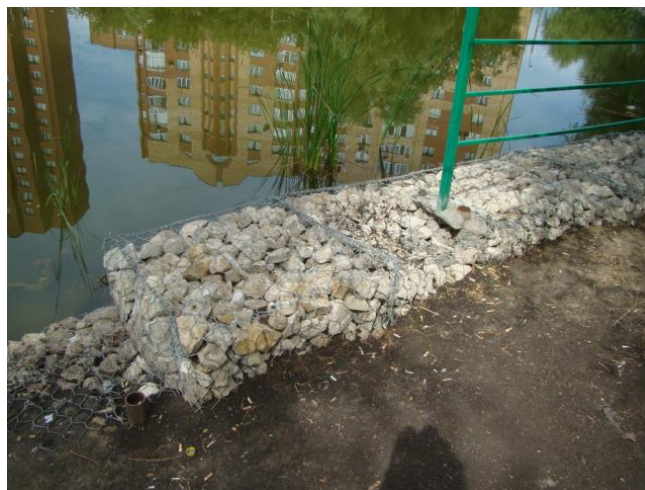
Fig. 1. Fragment of gabion structures
